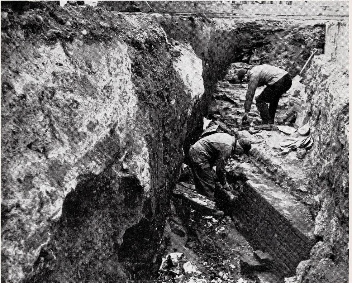
Fig. 7. Brick facing on wall of Fort Pitt between Grenadier and Flag Bastions. Test pit C.M. 3
