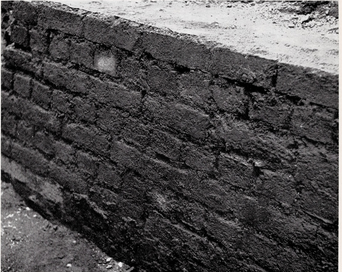
Fig. 9. Detail of brick facing of wall of Fort Pitt between Grenadier and Flag Bastions. Test pit C.M. 3
