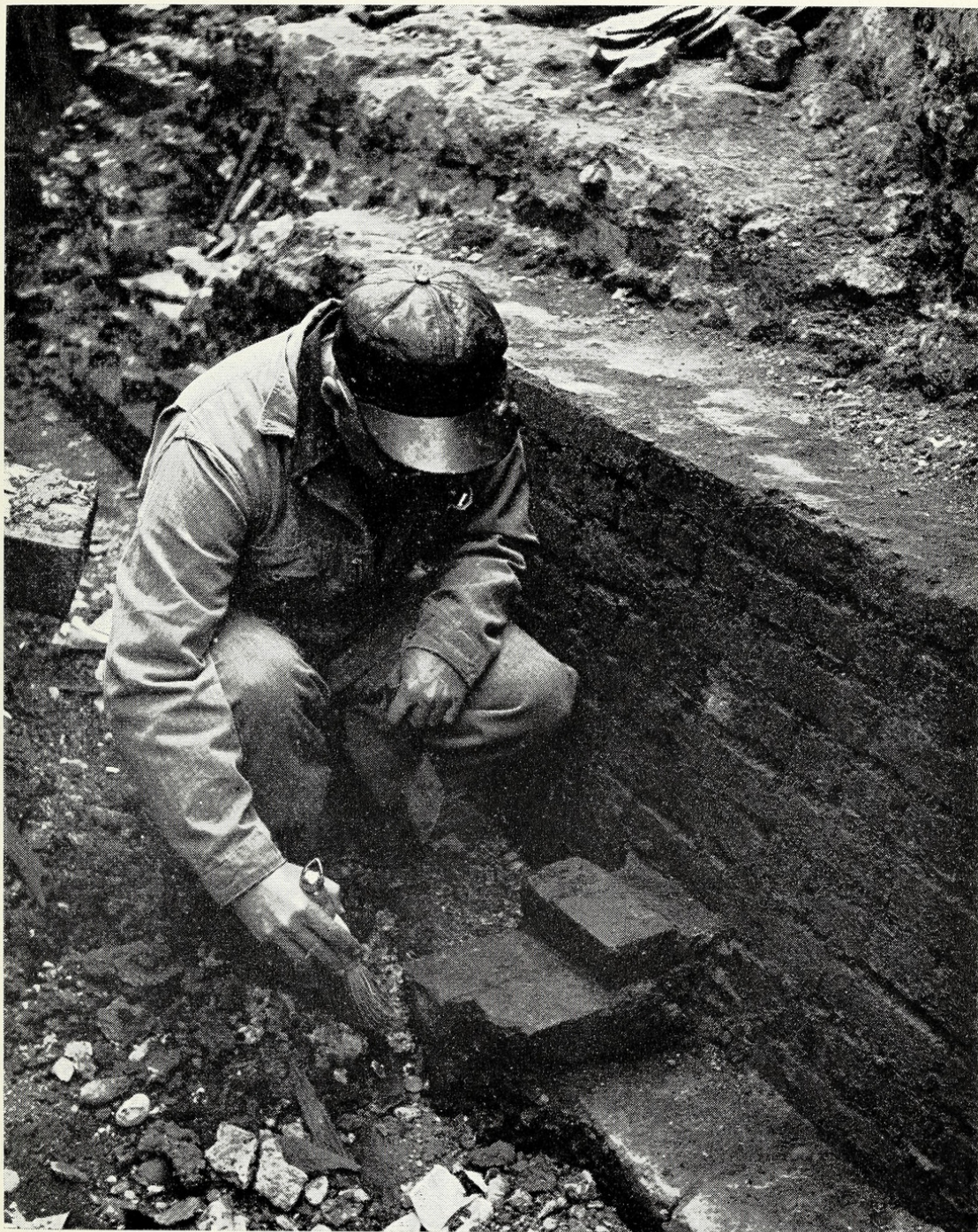
Fig. 8. Detail of brick facing at footer of wall of Fort Pitt between Grenadier and Flag Bastions. Test pit C.M. 3
