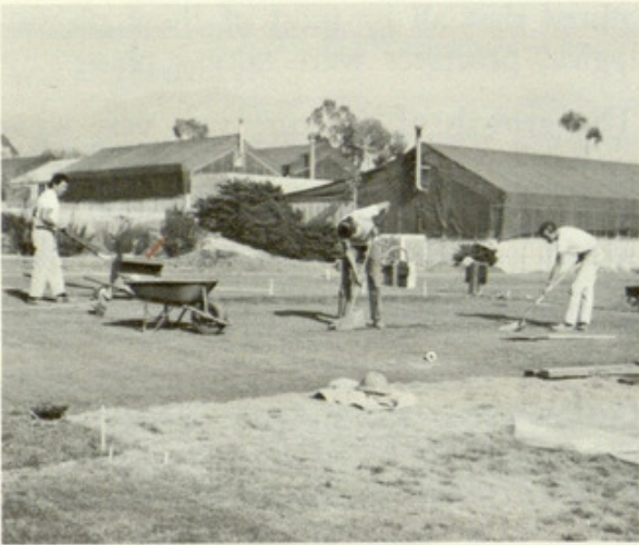
Backfilling trenches and firming soil over the cables was a tedious operation. Trenches totalled over 1/3 of a mile in length.
