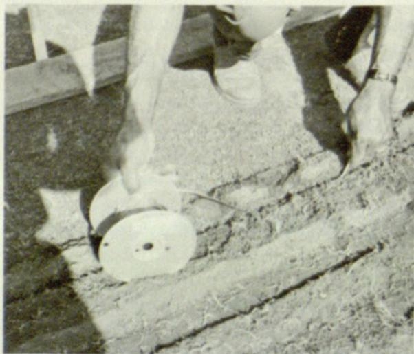
Cable being installed by hand into the trenches cut in bermudagrass sod.
