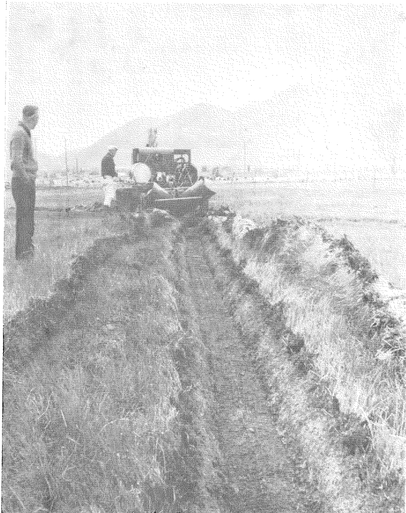
FIG. 1.—Ditch made by equipment described in text.
