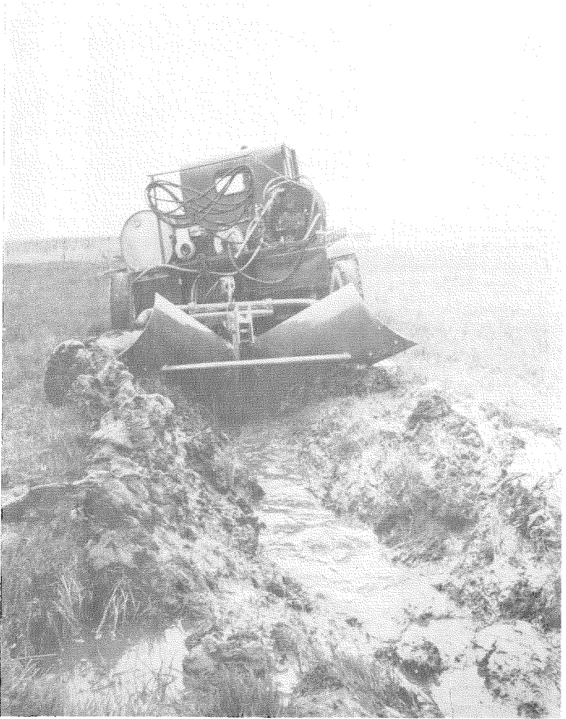
FIG. 2.—Spraying equipment installation on vehicle.
