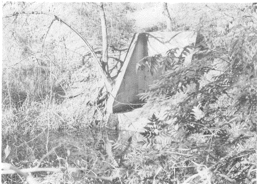
PLATE 1.—Storm sewer tunnel in the outskirts of Harlingen, Texas, from which St. Louis encephalitis isolates were obtained from six pools of Culex quinquefasciatus
