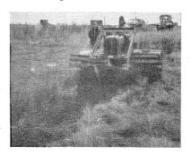
New salt marsh ditch cleaner, developed by R. C. Botsford, superintendent of the State Board of Mosquito Control, attacks a clogged ditch in a Connecticut marsh which, left uncleared, would make an excellent breeding place for mosquitoes.
